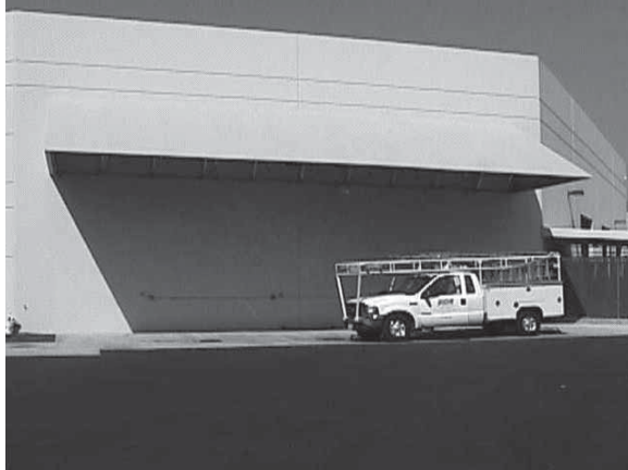
Awning integrated into building façade
